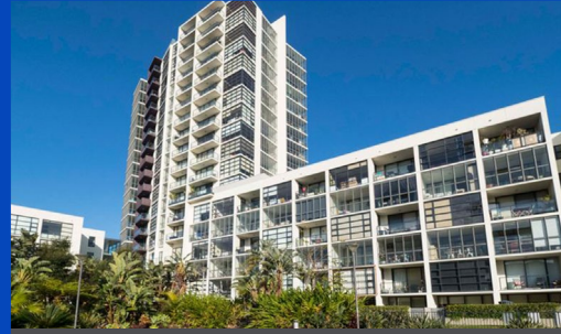
ZENIX APARTMENTS, ERSKINEVILLE Residential Remedial Project $10 MILLION
