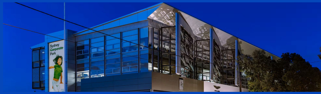
SYDNEY CORPORATE PARK Large Scale Commercial Cladding
